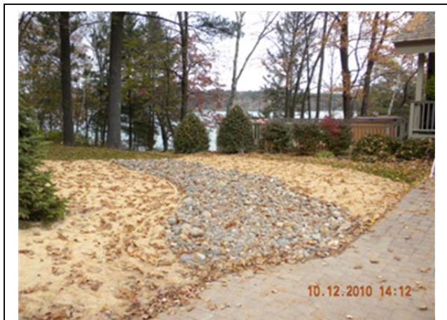
Rock infiltration between the driveway and the lake would prevent runoff, which carries nutrient and sediment, from entering Lake Owen.
